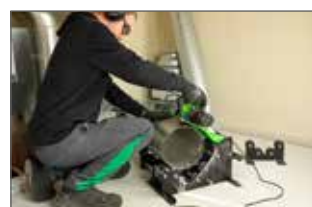
Quick cut of ventilation pipes
